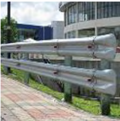
Figure 4: W-Beam Guardrail
