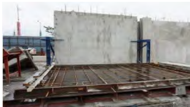
2. Insert the reinforcement & piping.
