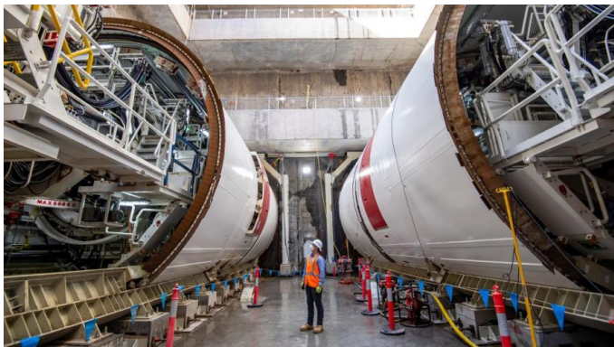
Figure 1: TBM Betty (left) and TBM Dorothy (right)
