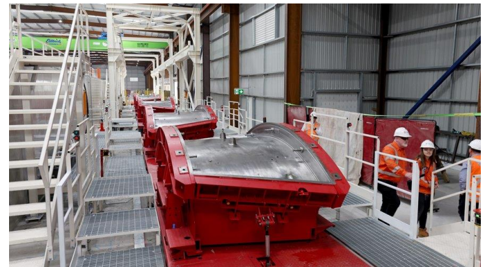
Figure 2: Precast concrete production floor
