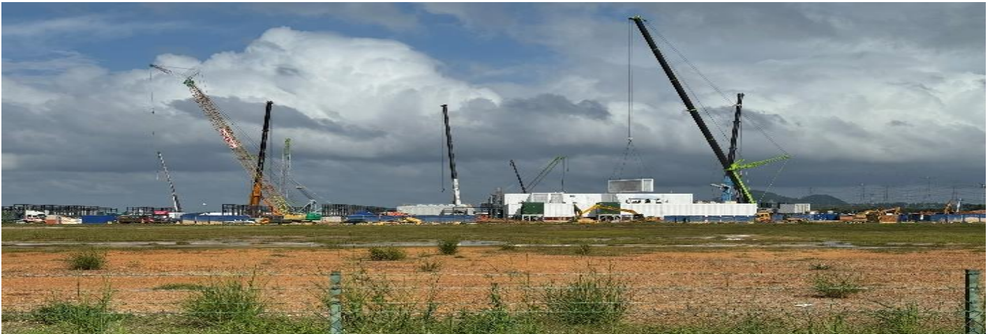
Figure 3: SunCon's K2 data centre project
