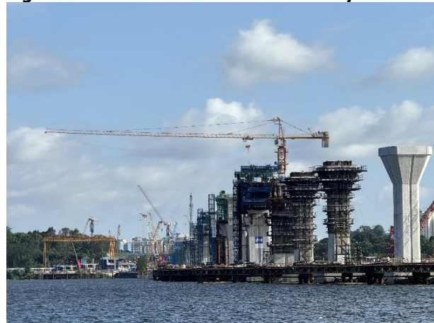
Figure 2: Marine viaducts constructed by CCCC
