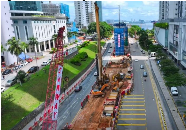
Figure 1: SunCon's RTS job in Jalan Tun Abdul Razak
