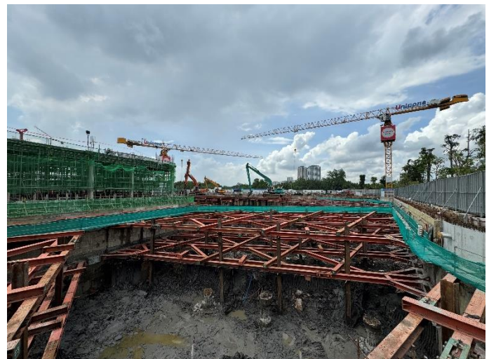
Figure 2: Construction ongoing at the Eaton Park site
